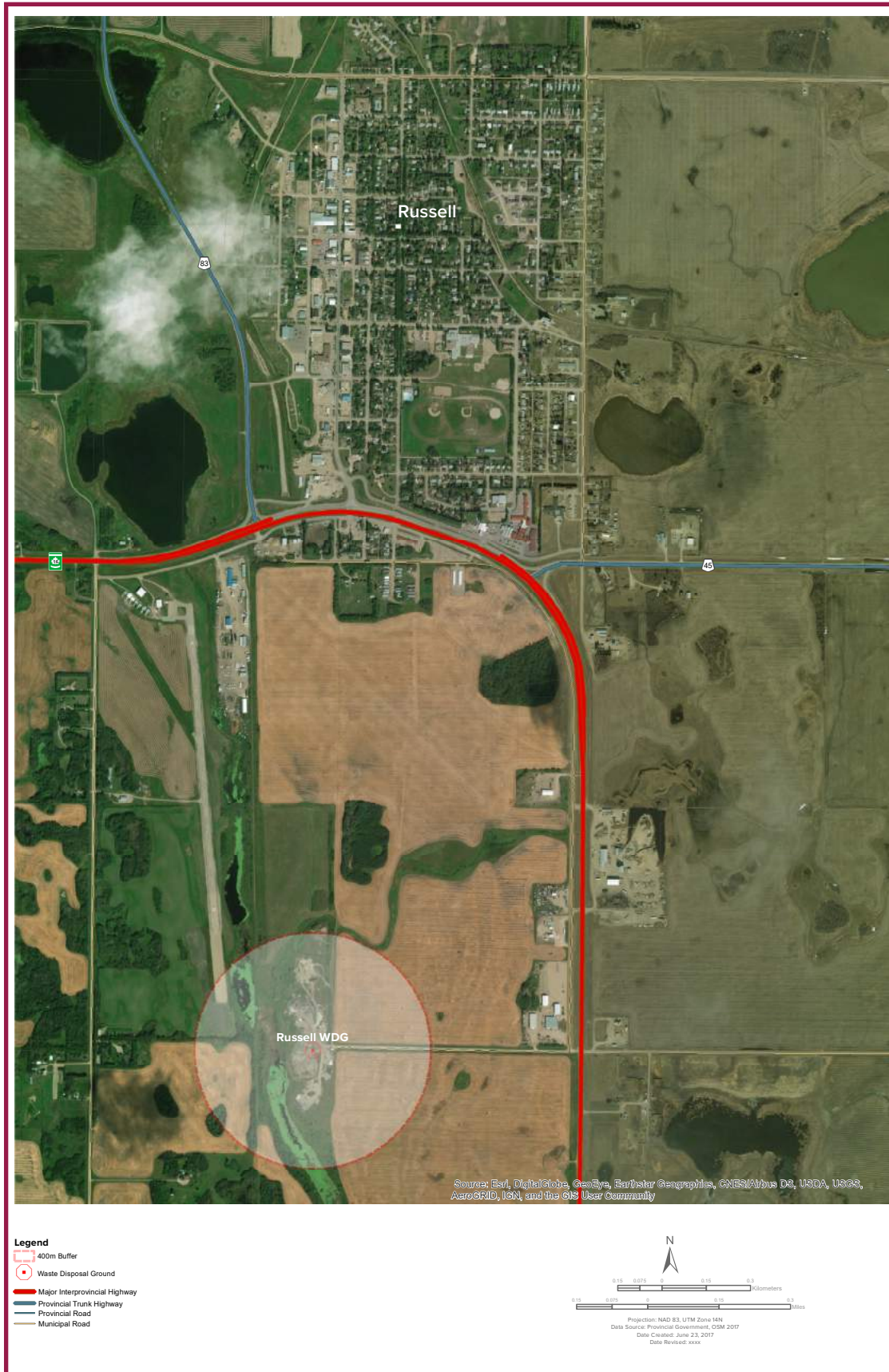
Figure 23: Russell Waste Disposal Grounds and Buffer Area
